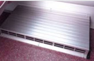
Air return grille of sub heater
